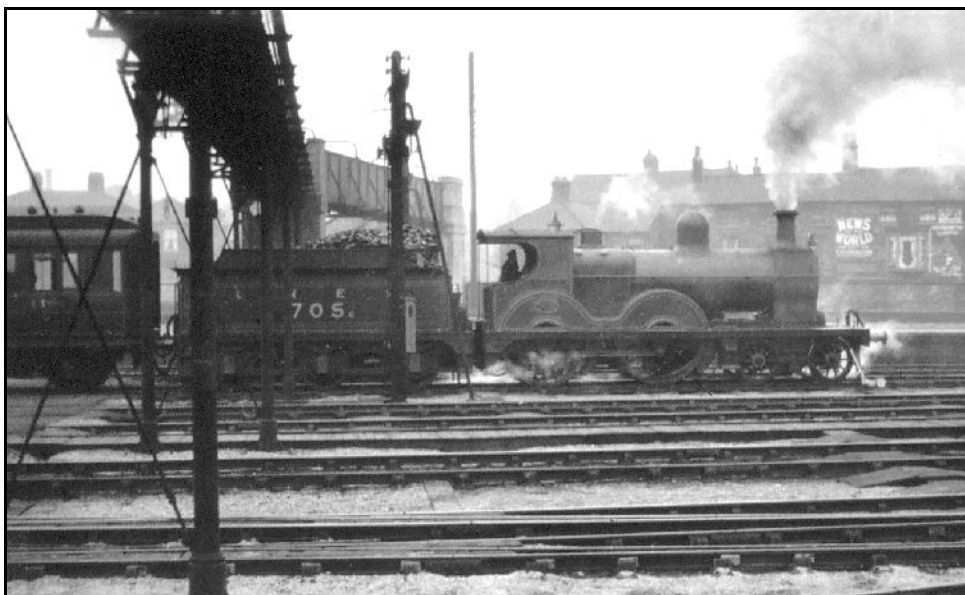
Class D7 4-4-0 no.705c departs from the east end of Lincoln Central in 1924. Formerly GCR class 2, it was designed by Parker for the MSLR. The prototype, no.561, was built by Kitson and displayed at the Manchester Exhibition in 1887. For this reason, the class 2 was also known as the "Class 561". No.705 was built in 1892 and survived until 1933.
