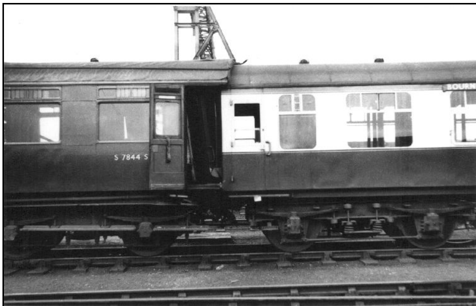
The damage caused to the ex-SR restaurant car is evident in this photograph taken by David Sutcliffe on the morning after the accident. photo: D.M.Sutcliffe
