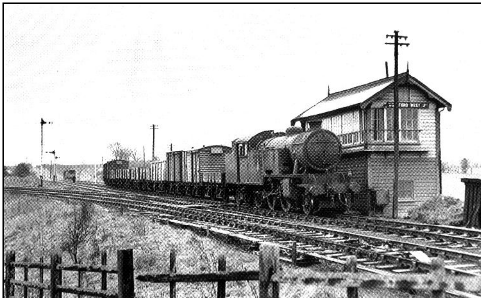
BR class L1 2-6-4T no.67789 with the 2.20pm transfer freight from Woodford Halse at Woodford West Junction. The train is being backed into the sidings that once formed the south-to-west spur. The line coming in from the left is from Woodford North Junction. The bridges visible in the background carry a road over the SA&MJ and the south-to-west spur. The GC main line passes under the SA&MJ at a point beyond the bridges. Byfield station is directly behind the photographer. Date is unknown.
